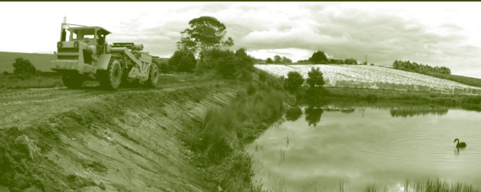
Repairing the dam wall
